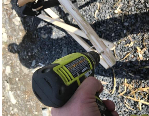
Drill holes with 1/2 inch bit
